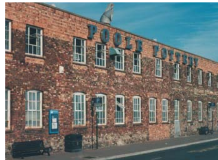
Exterior of the Poole Pottery building facing Poole Harbour.
