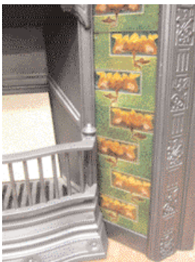
Tiles change a fireplace dramatically. The original Arts & Crafts tiles here are in good condition, but will cost 3-4 times as much as a set of similar reproduction tiles. Image: www.oldfireplaces.co.uk .
