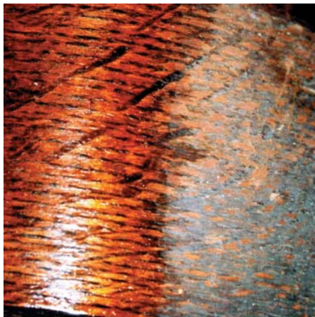
Fig 2. The oak veneer of this Napoleon Hat clock was in a terrible condition. The half-restored case was first oiled to bring out the grain and then French polished. This is easy to do and the results are a striking improvement.
